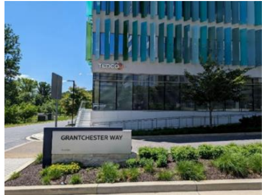
View of building driving down Grantchester Way
